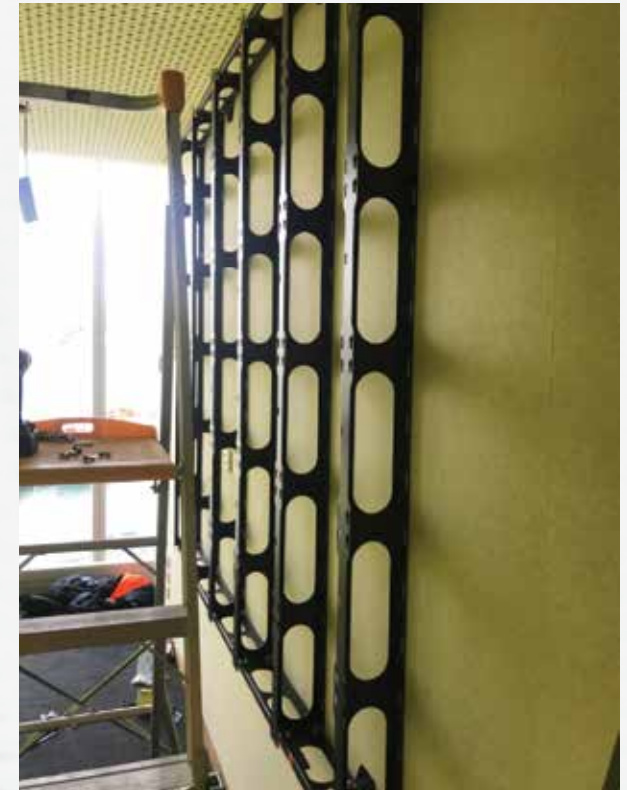
Wall Mount Bracket with all framework in position.
